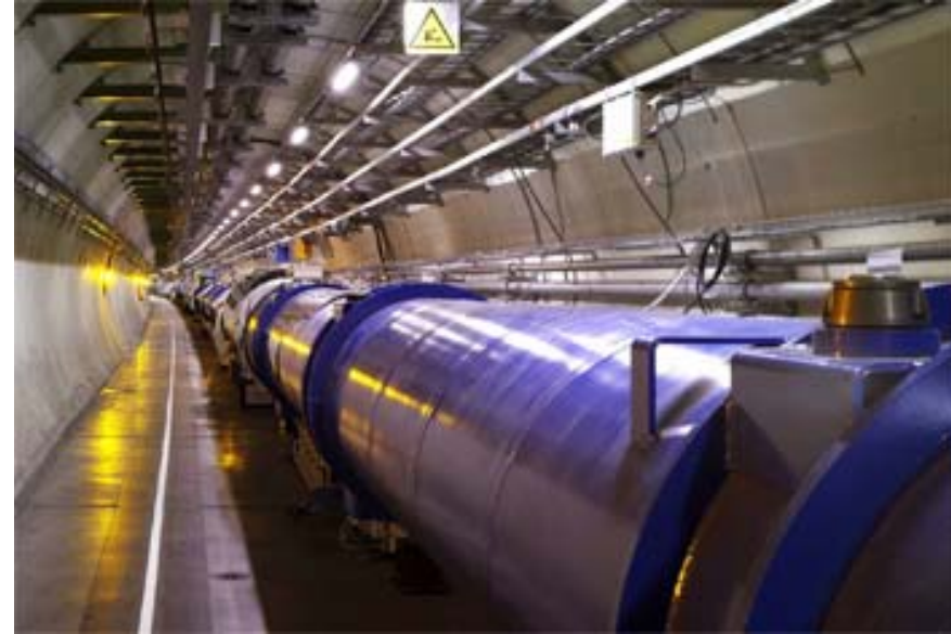
Inside the tunnel.
